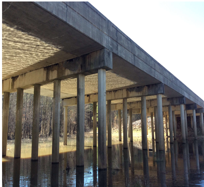
PHOTO 4 Description Spalls at bent 7,6,5
