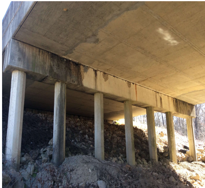
PHOTO 1 Description BT 18 spall 8 LF
