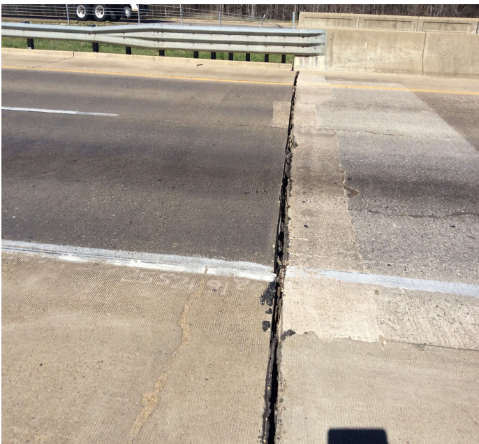
PHOTO 1 Description CONSTRUCTION JOINTS OVER BENTS JOINT MATERIAL IS COMING OUT OF JOINTS AT VARIOUS LOCATIONS
