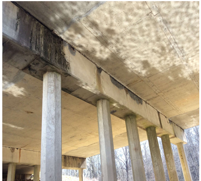
PHOTO 2 Description BT 17 spall 13 LF
